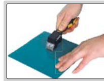
step 1: make grid cutting on surface
